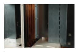
The 4 pole busbar system ready to accept the circuit breaker.
