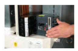
The circuit breaker is placed in the panelboard and pushed up to the busbars. 1P, 2P, 3P and 4 pole breakers may be mixed in any order on the busbars.
