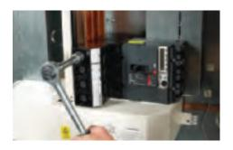
The connections to the busbars are tightened until the tops of the connection bolts shear off. This ensures that the correct torque has been applied to the connections.
