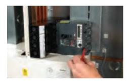
The circuit breaker fixing screw is fitted and tightened to retain the breaker in the board.
