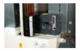
The circuit breaker is now mechanically & electrically connected in the panel board. It is now ready for the outgoing cables.
